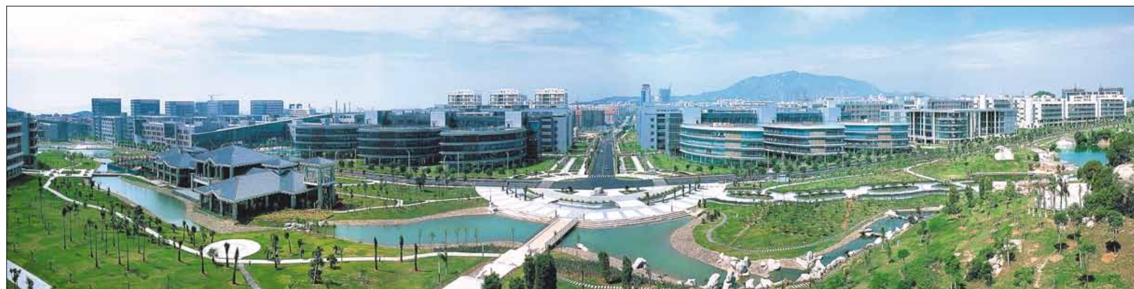
The second phase of the Software Park at the Xiamen National Torch Hi-Tech Industry Development Zone, or Torch Hi-Tech Zone for short. PROVIDED TO CHINA DAILY
