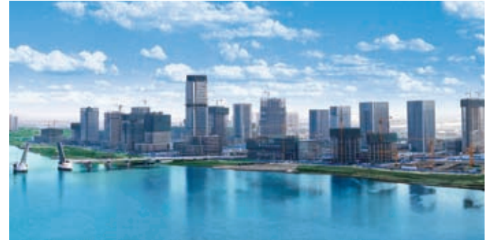
Xianluowan Business Area under Construction
