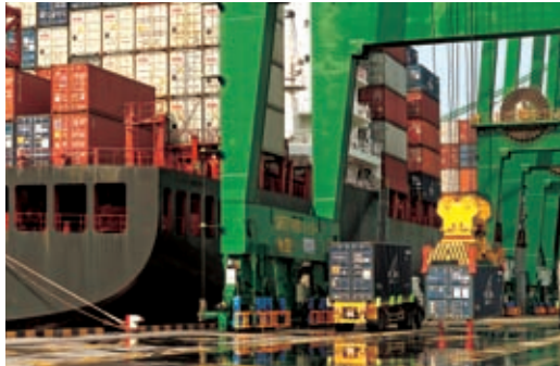
Tianjin Port Container Wharf
