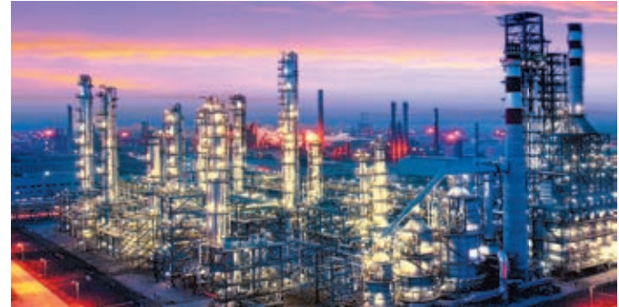
Sinopec Tianjin Million-ton Ethylene Refining-Chemical Integration Project
