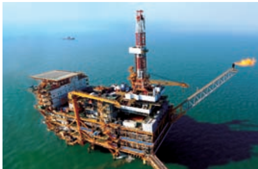
Offshore Oil Drilling Platform of Bohai Oil Field
