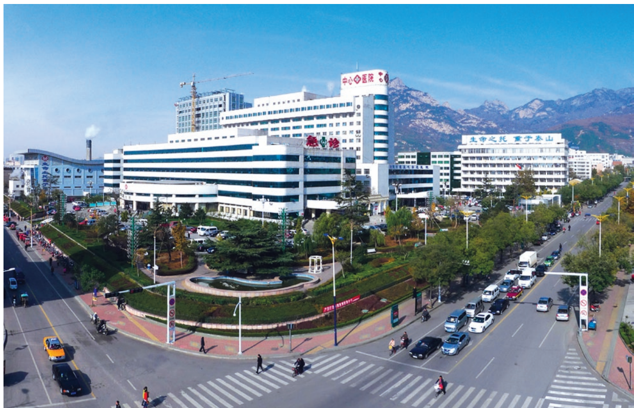
Tai'an Center Hospital
