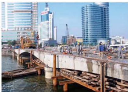
Guangchang Bridge In demolition in 2007
