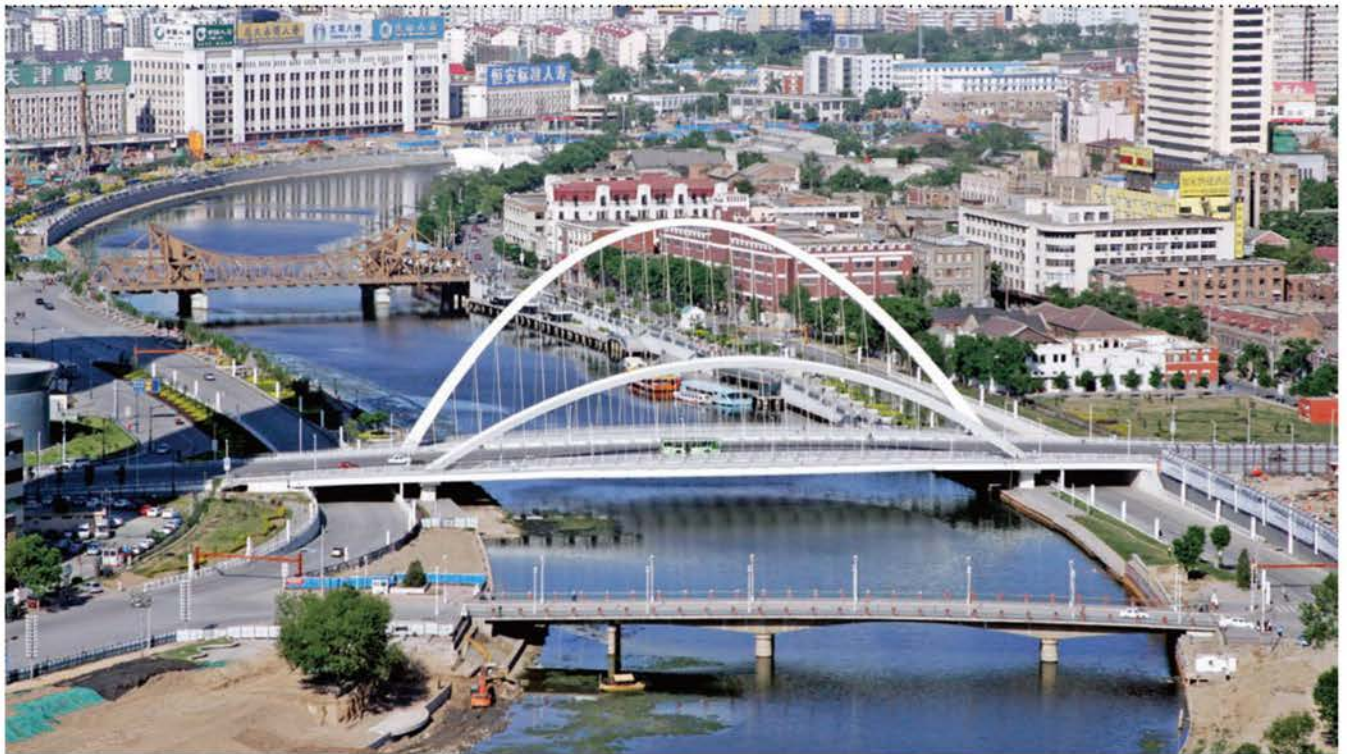
Guangchang Bridge and Dagu Bridge
