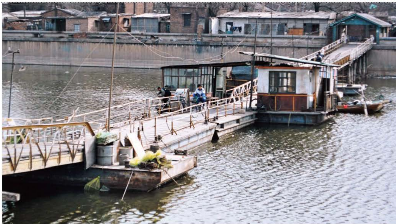
Beikai Floating Bridge
