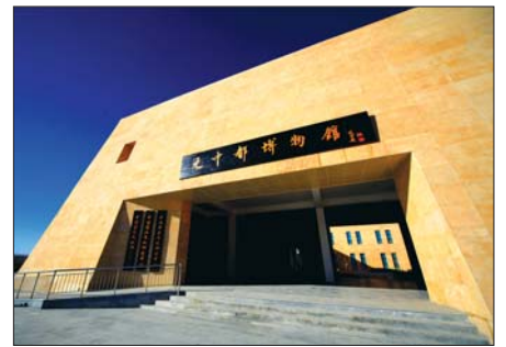
The newly built 80 million yuan Zhongdu museum covering the Yuan Dynasty (1271-1368) will house relics and serve as a place to study the imperial architecture of the Mongol empire as well as nomadic culture.
