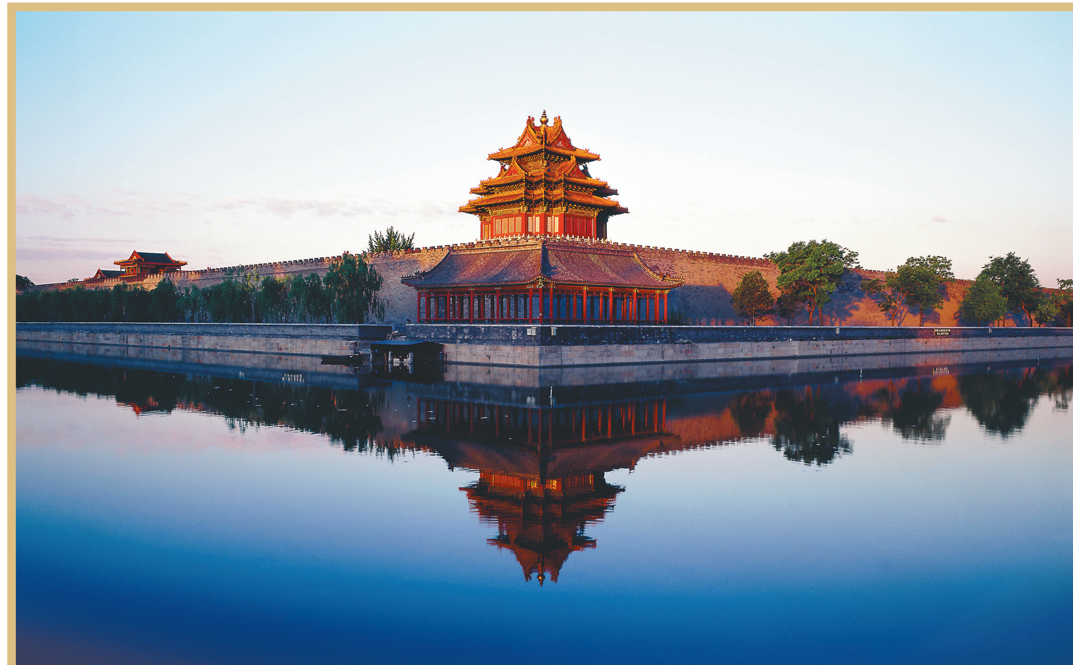
Turrets are an important part of the Forbidden City's defense system. Their complex structure is usually described as "nine beams, 18 pillars and 72 ridges".
