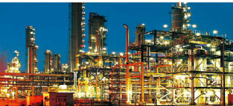
Sinopec One-million-ton Ethylene Cracker in Tianjin
