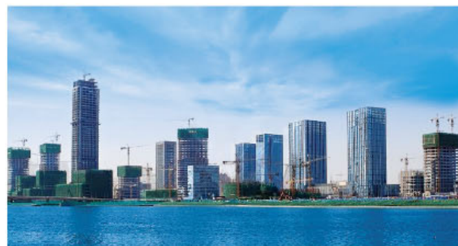
Xiangluowan Business District under Construction
