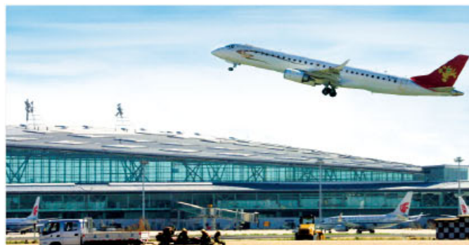
Tianjin Binhai International Airport
