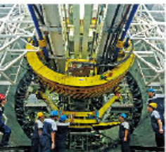
The Subway Shield Tunneling is Crossing the Haihe River
