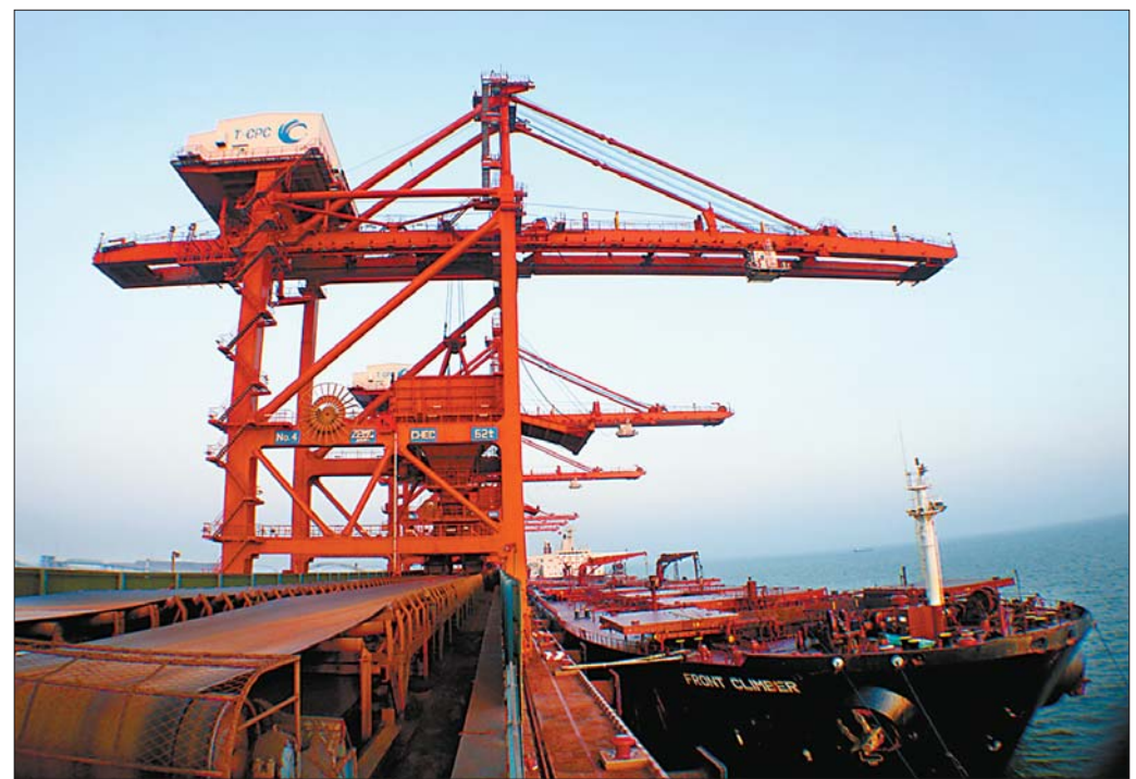
A wharf in Tangshan Bay, Hebei province.
