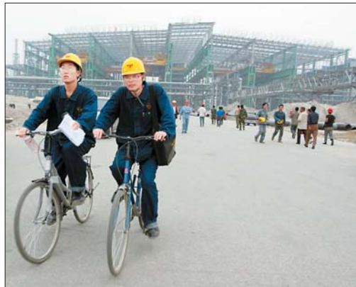
Workers at a construction site in Caofeidian, Tangshan, Hebei province.
