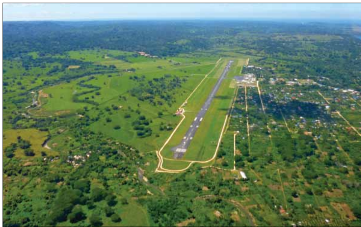
The international airport at Port Vila is receiving an upgrade. PHOTOS PROVIDED TO CHINA DAILY
