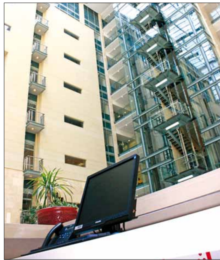
A section of ATW's glass-roofed atrium, which allows natural sunlight in.
