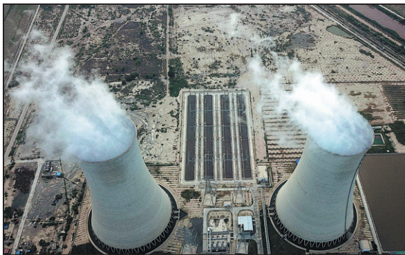
Two cooling towers are seen in the Sahiwal Thermal Power Plant in the Pakistani city of that name in August. The coal-fired plant, which generated 9 billion kWh of electricity in 2018, is among a number of energy projects along the China-Pakistan Economic Corridor. PHOTO BY XINHUA
