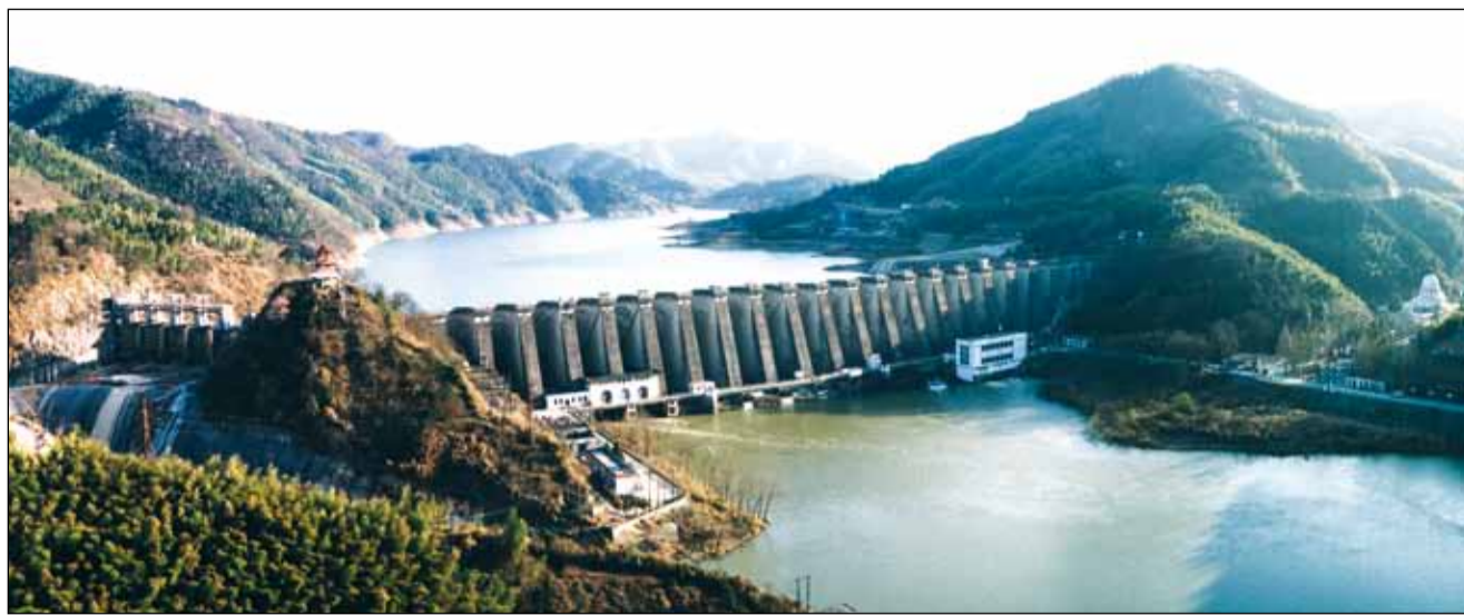
Foziling Reservoir, one of six major reservoirs in Lu'an, Anhui province, a major source of hydroelectric power for the area.
