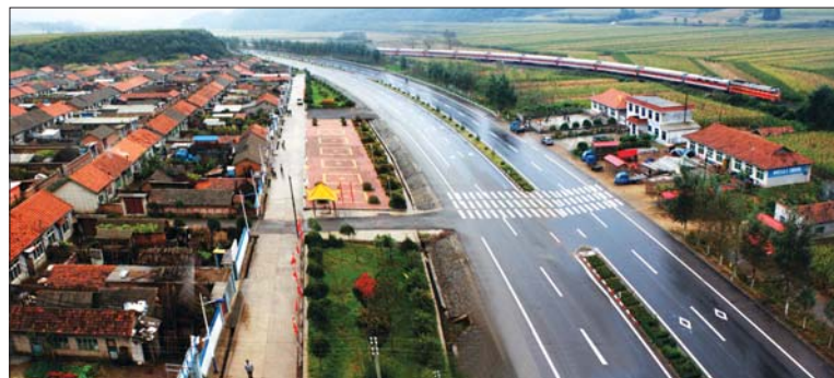
Urban road construction has been prioritized in the cold northwestern province.
