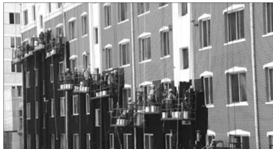
Workers restore the exterior of old residential buildings in Changchun, Jilin.
