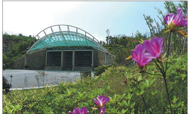
Foxconn's data center in Guian has 6,000 servers. LI FENG / FOR CHINA DAILY
