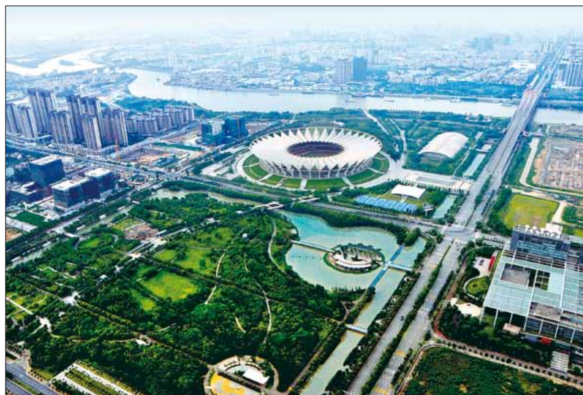
The sound eco-system is factored in the decision to establish the industrial service zone in Foshan.
