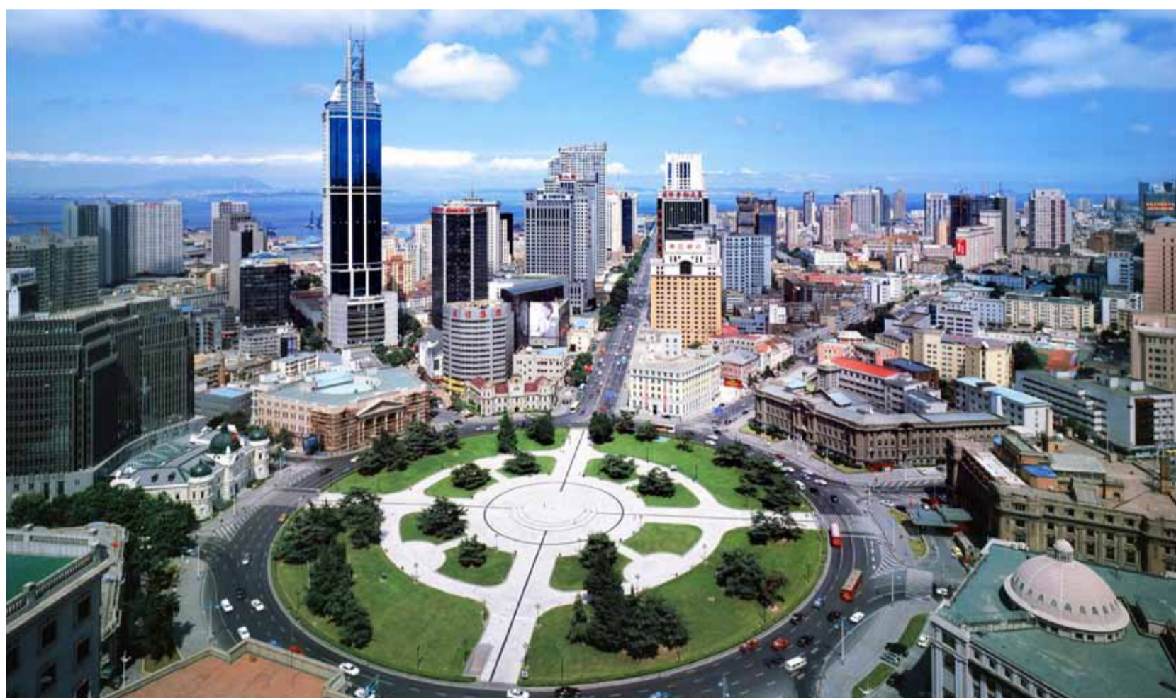
The area surrounding the Zhongshan Square is the central business district of the city.
