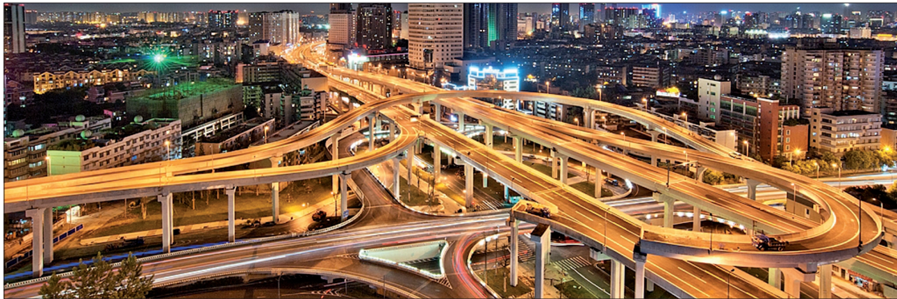
Yingmenkou flyover, a landmark on the second ring road in Chengdu.
