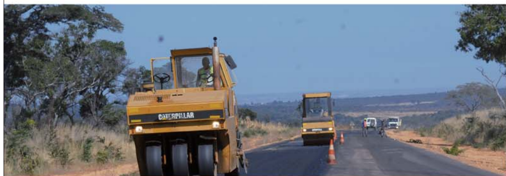
Construction of a road in Menongue
