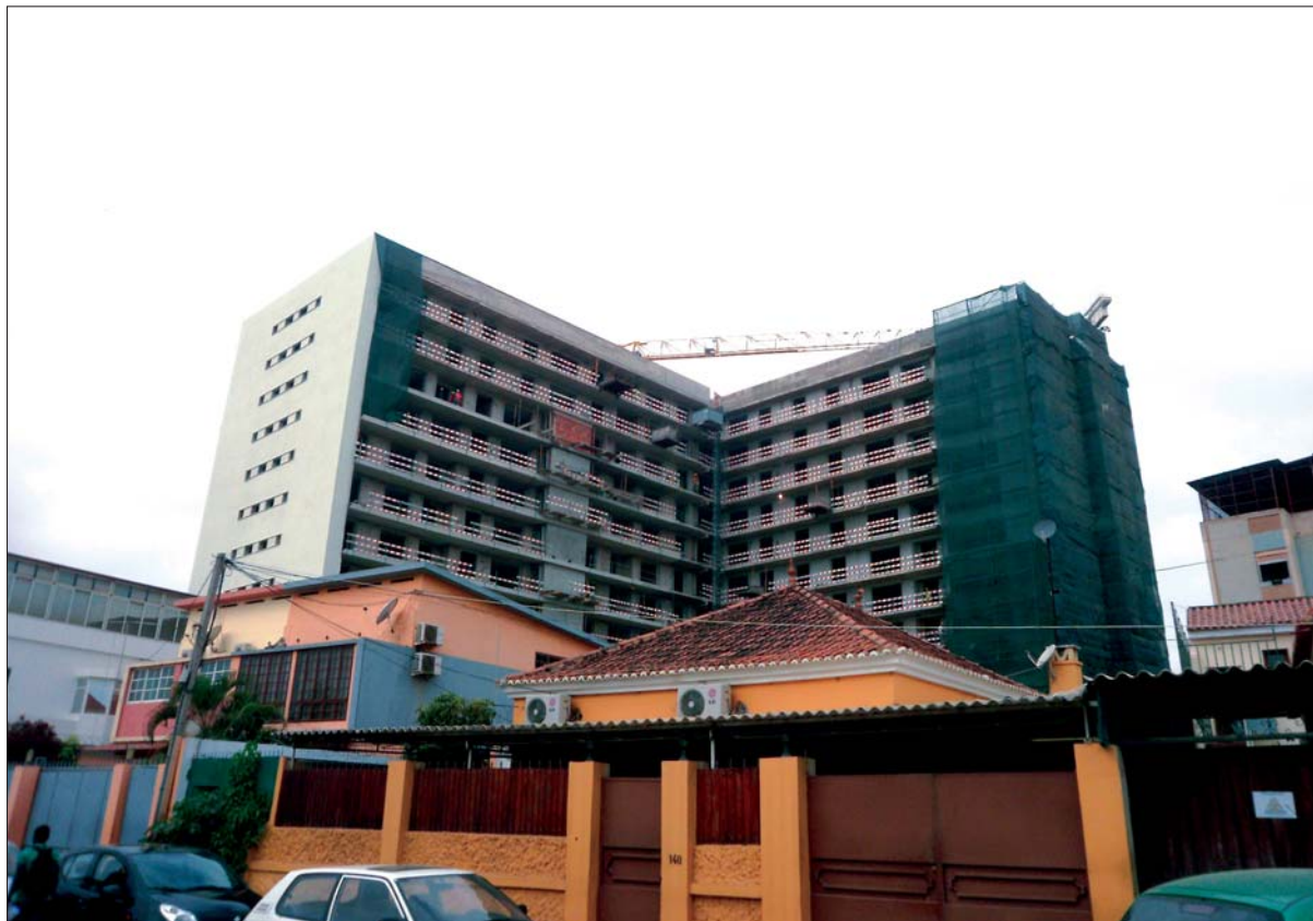
One of Edifer's buildings in Luanda, capital city of Angola.
