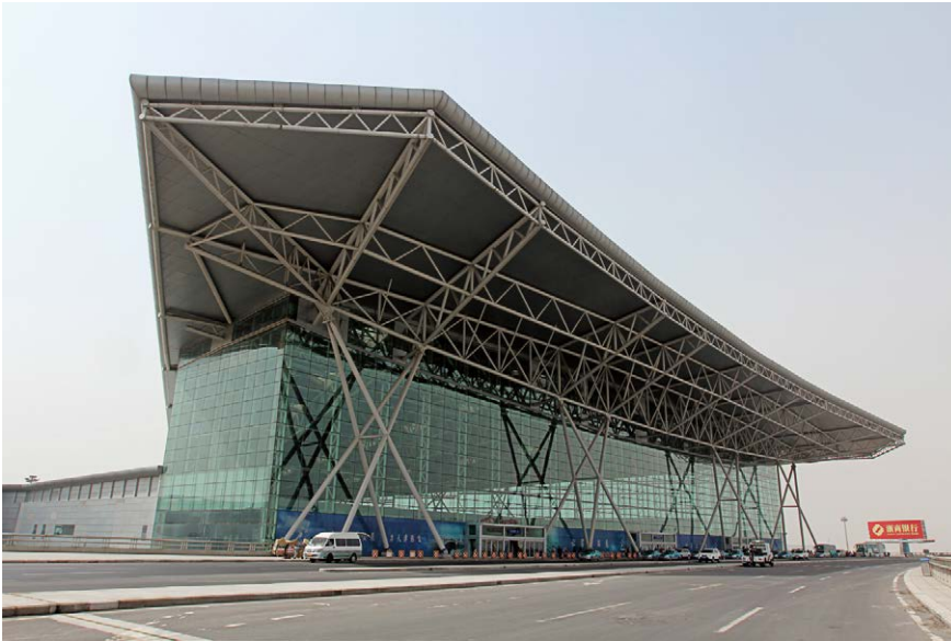
Tianjin Binhai International Airport
