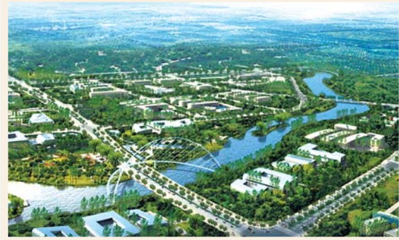
Aerial view of hi-tech industry park
